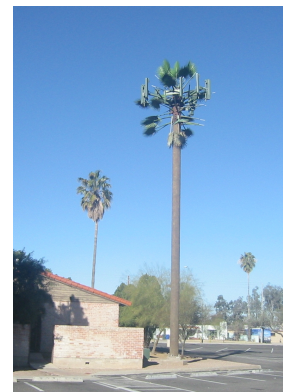
Telephone site concealed as a palm tree.
