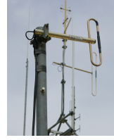
Folded dipole antenna
