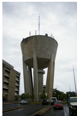
A water tower in Palmerston, Northern Territory with radio broadcasting and communications antennas.
