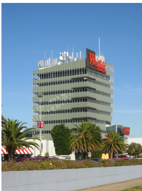
A building rooftop supporting numerous dish and sectored mobile telecommunications antennas (Doncaster, Victoria, Australia).
