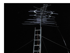
A US multiband "aerial" TV antenna.
