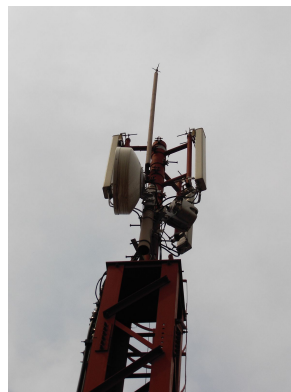
A three-sector telephone site in Mexico City.
